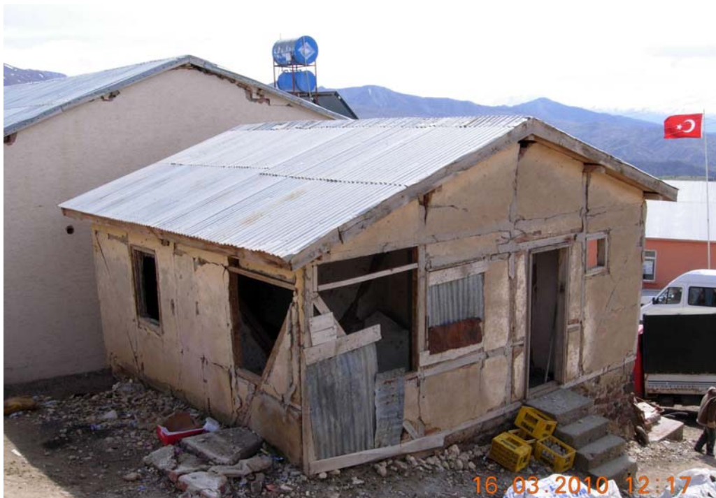
Figure 57: Refractory brick houses built after 1971 Bingol earthquake, Okcular
