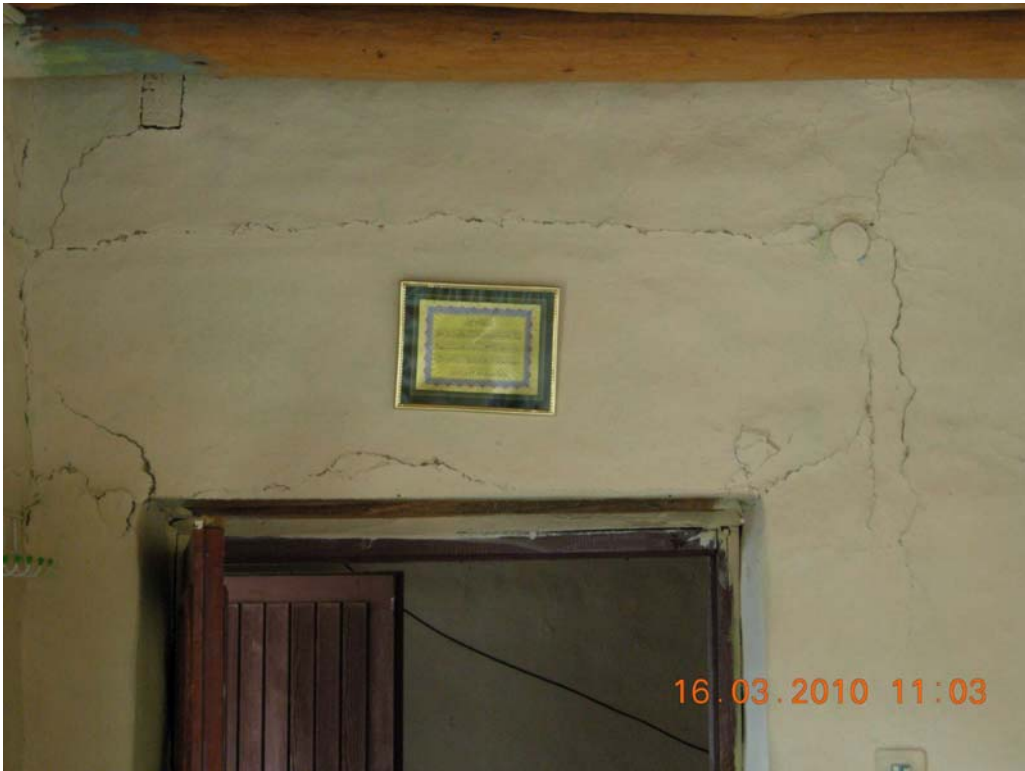
Figure 91: Inside view of two storey soil brick house in Kökan-Bayramyazı-5
