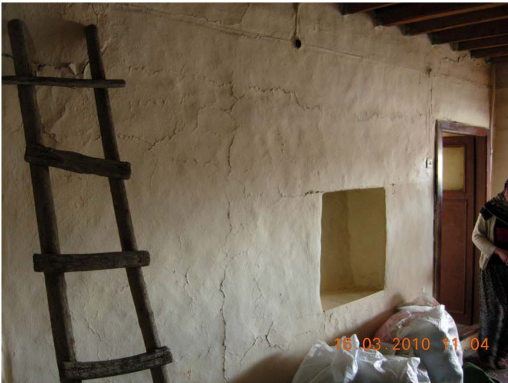
Figure 94: Inside view of two storey soil brick house in Kökan-Bayramyazi-8
