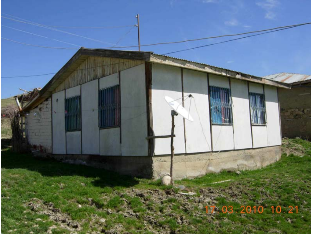
Figure 61: Prefabricated panel houses built after 1971 Bingol earthquake, still in use, Incedal village
