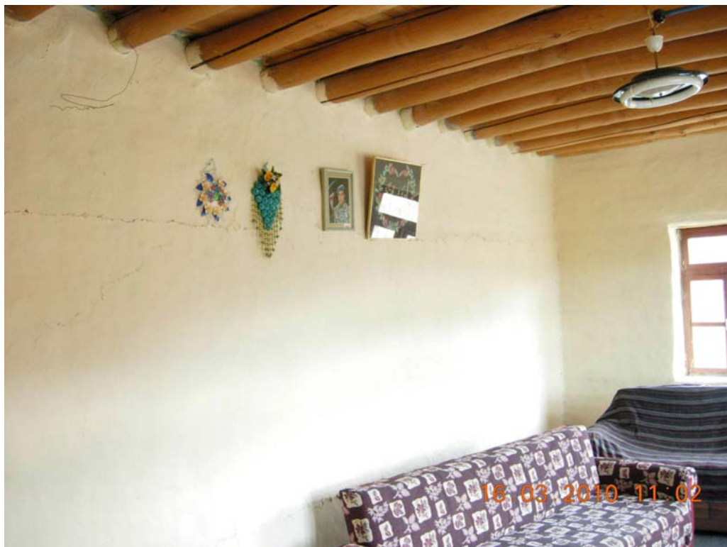
Figure 88: Inside view of two storey soil brick house in Kökan-Bayramyazı-2
