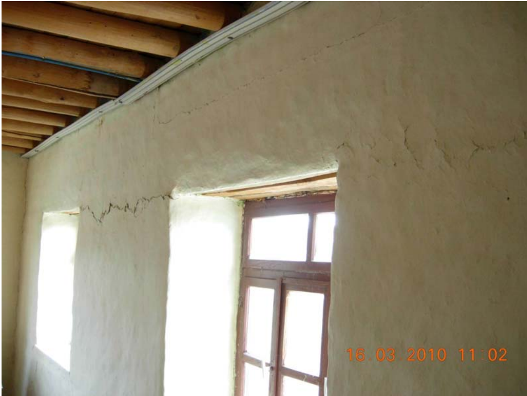
Figure 89: Inside view of two storey soil brick house in Kökan-Bayramyazı-3
