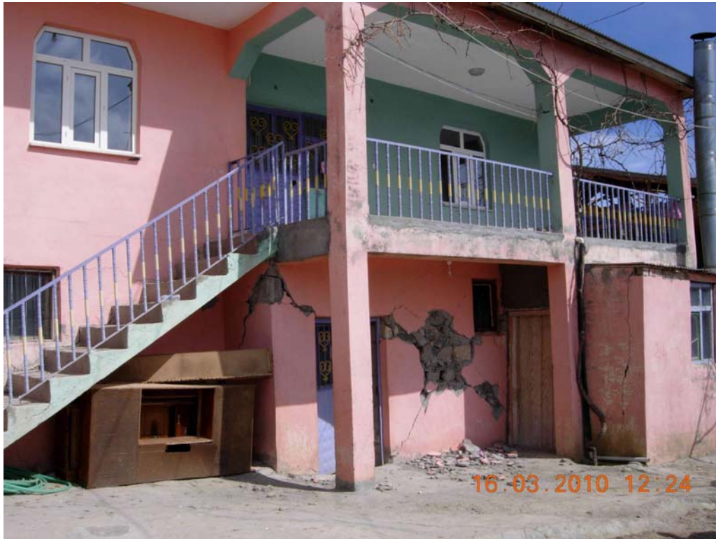
Figure 39: Outside view of two storeys mixed structural system, Okcular village
