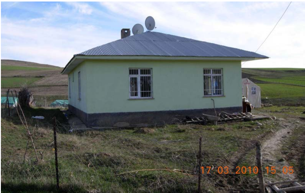
Figure 66: RC house, built by government, after 2003 Bingol earthquake, Tabanözü village
