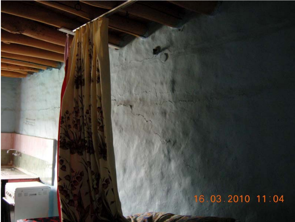
Figure 95: Inside view of two storey soil brick house in Kökan-Bayramyazı-9
