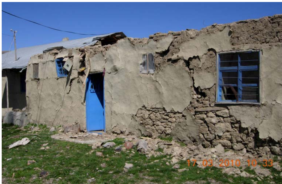
Figure 18: One storey soil brick house in Incedal village-side view 1 (bottom part of the house, below window level is built with stones)
