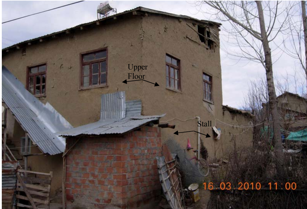
Figure 87: Outside view of two storey soil brick house in Kökan-Bayramyazı-1
