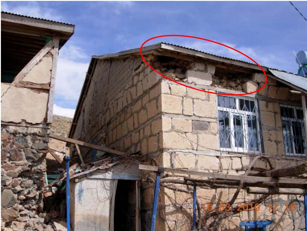
Figure 28: Upper floor of two storey light stone house, with a stall as ground floor, Okcular village
