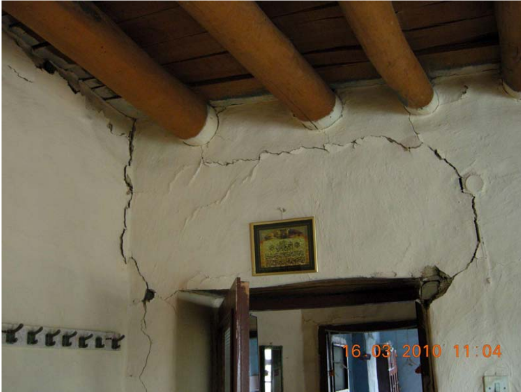
Figure 93: Inside view of two storey soil brick house in Kökan-Bayramyazi-7
