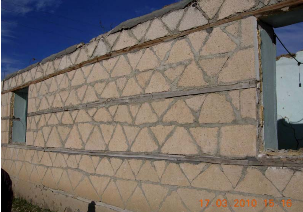
Figure 85: Single example of properly arranged, layered, triangular shaped, one story house, inside walls are soil bricks, Tabanözü village
