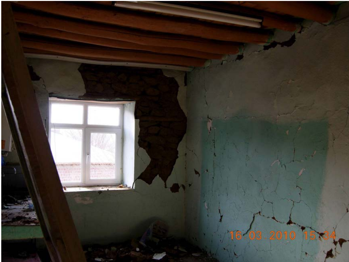
Figure 38: Two storey heavy stone house, inside view, Beyhani
