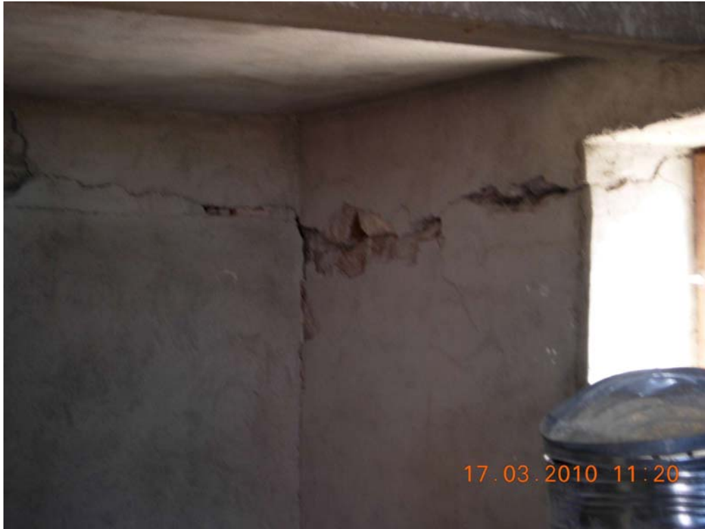
Figure 45: Inside view of two storeys mixed structural system, RC beam, RC slab, heavy stone wall, Okular village
