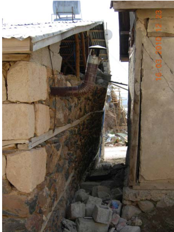
Figure 74: Out of plane failure due to length of wall in two story stone house, Okcular village
