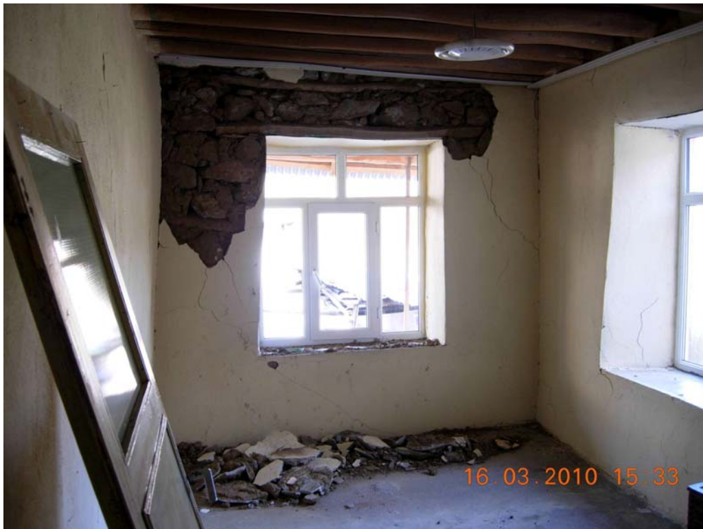
Figure 37: Two storey heavy stone house, inside view, Beyhani
