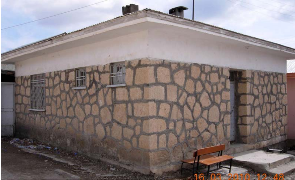
Figure 26: One story typical school building, Okcular village
