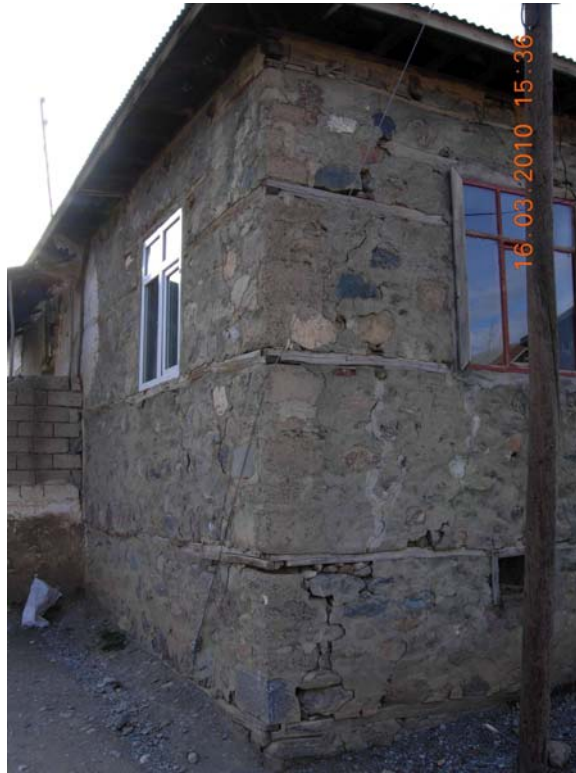
Figure 36: Two storey heavy stone house, side view, Beyhani
