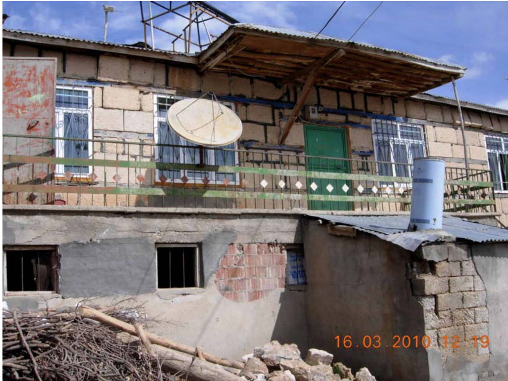
Figure 30: Two storey light stone house, with a stall as ground floor, Okcular village
