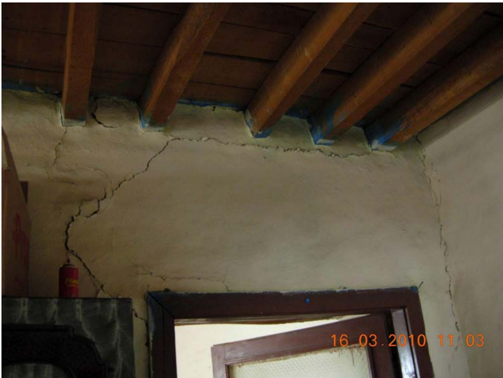
Figure 92: Inside view of two storey soil brick house in Kökan-Bayramyazı-6
