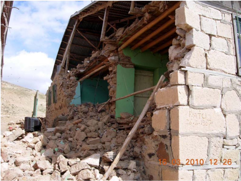
Figure 32: Two storey light stone house, constructed in 1987, Okcular village
