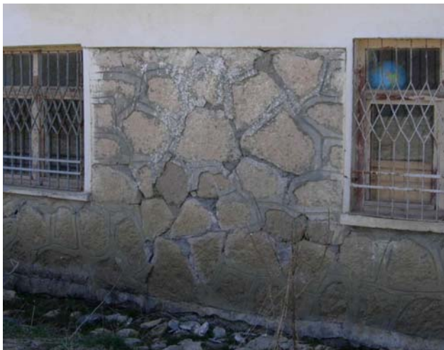
Figure 84: Improperly arranged stone walls, İncedal village
