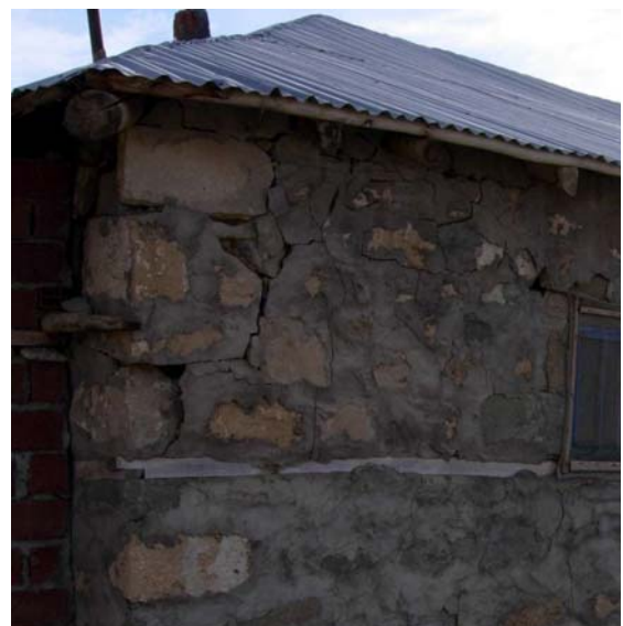
Figure 84: Improperly arranged stone walls, İncedal village
