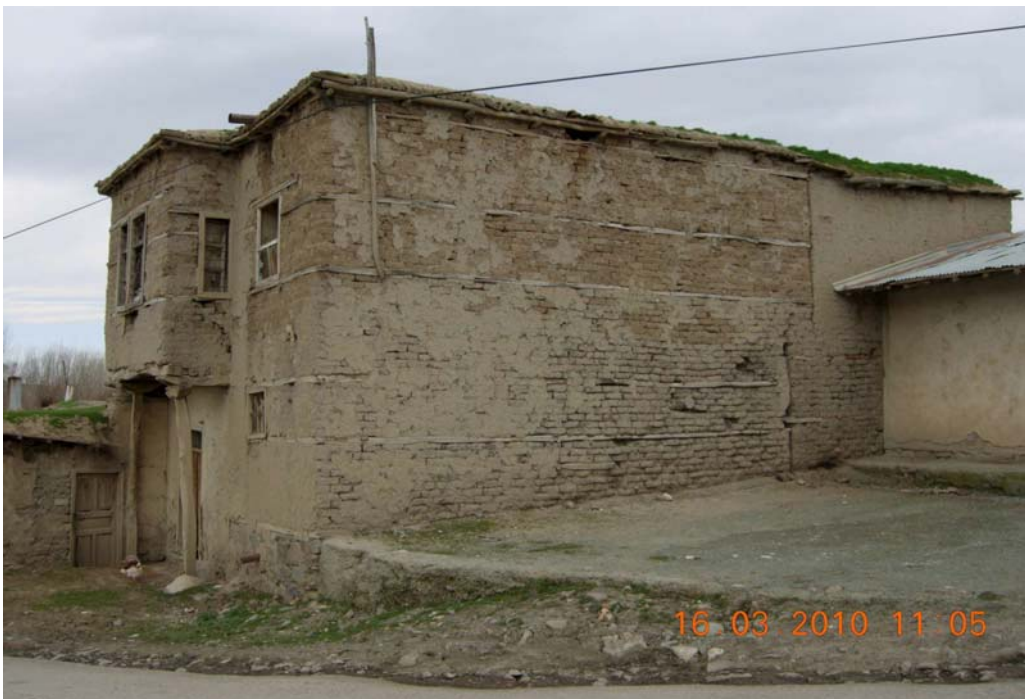
Figure 20: Outside view of two storey soil brick house in Kökan-Bayramyazi
