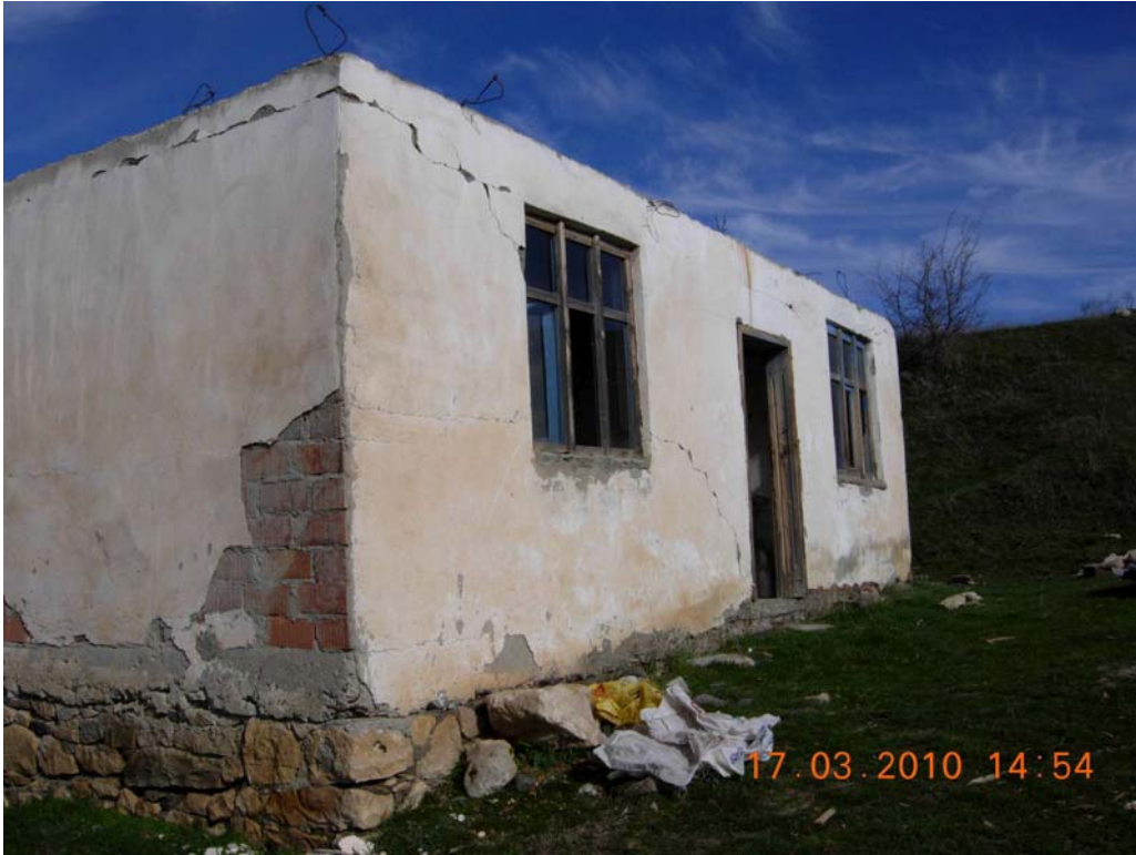
Figure 47: One storey house, built with infill bricks, Aşağıkanathı village
