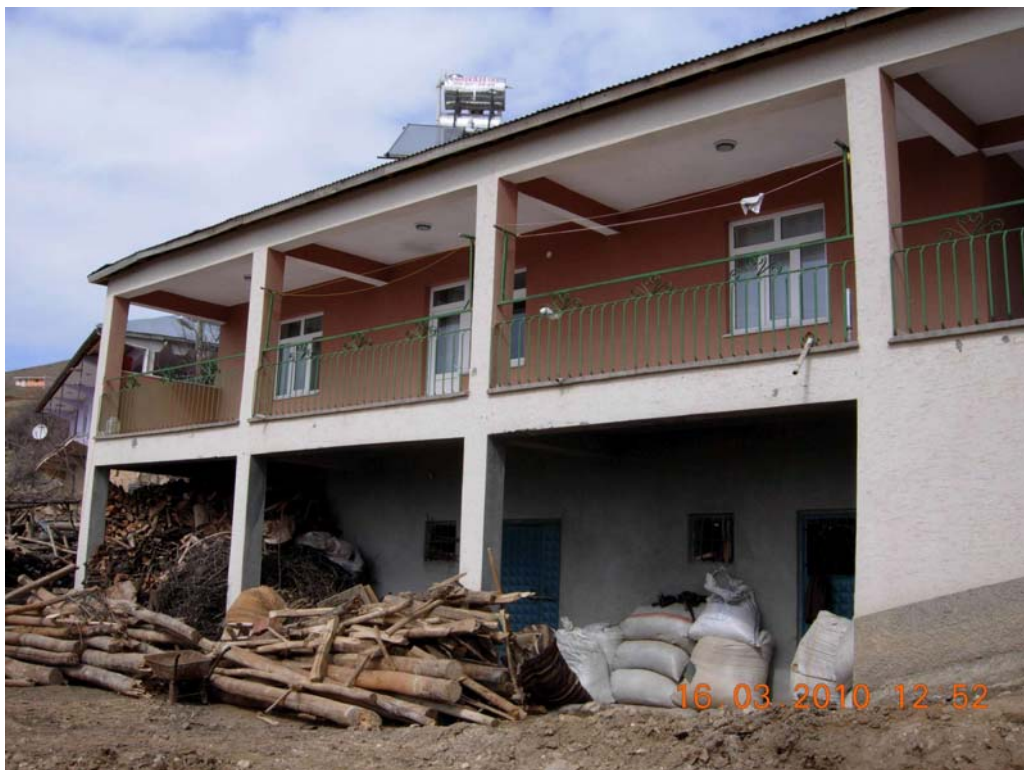
Figure 64: RC house, without any damage in beam-column joints, Okcular village
