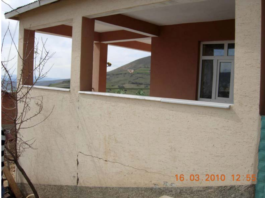
Figure 63: RC house, without any damage in beam-column joints, Okcular village
