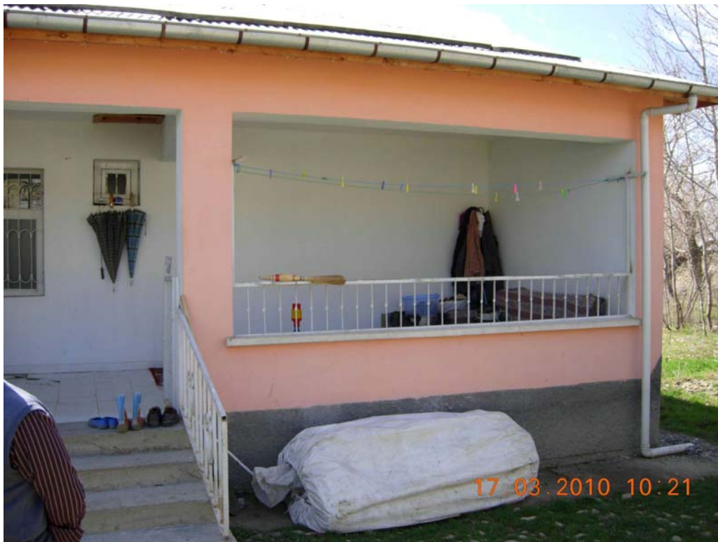
Figure 67: RC house, built by government, after 2003 Bingol earthquake, Incedal village
