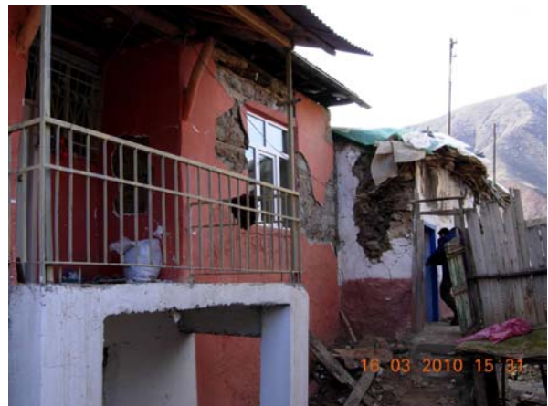
Figure 83: Wide cracks around openings, Beyhan-Palu
