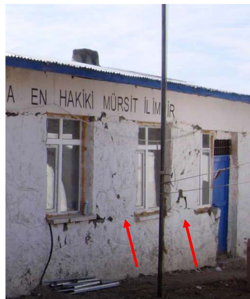
Figure 81: Wide cracks following the mortar, school building side view, Kayalık village
