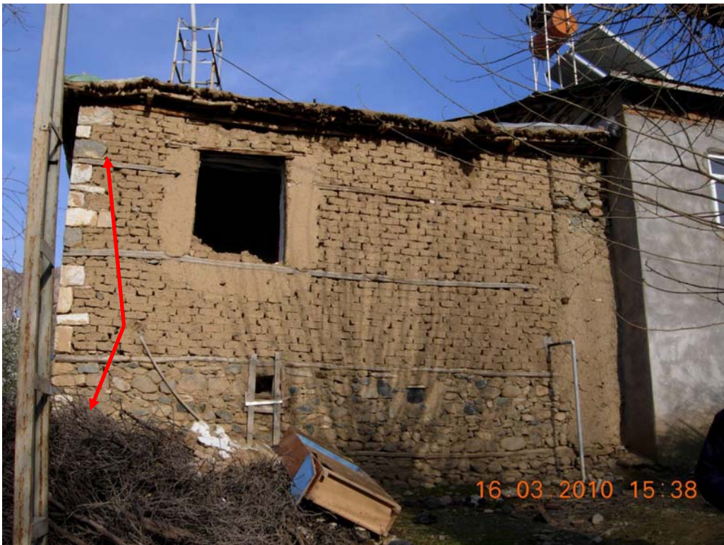
Figure 24: Two storey soil brick house with a stall in the ground floor (only lintel application ever seen in that area), side view, Beyhani
