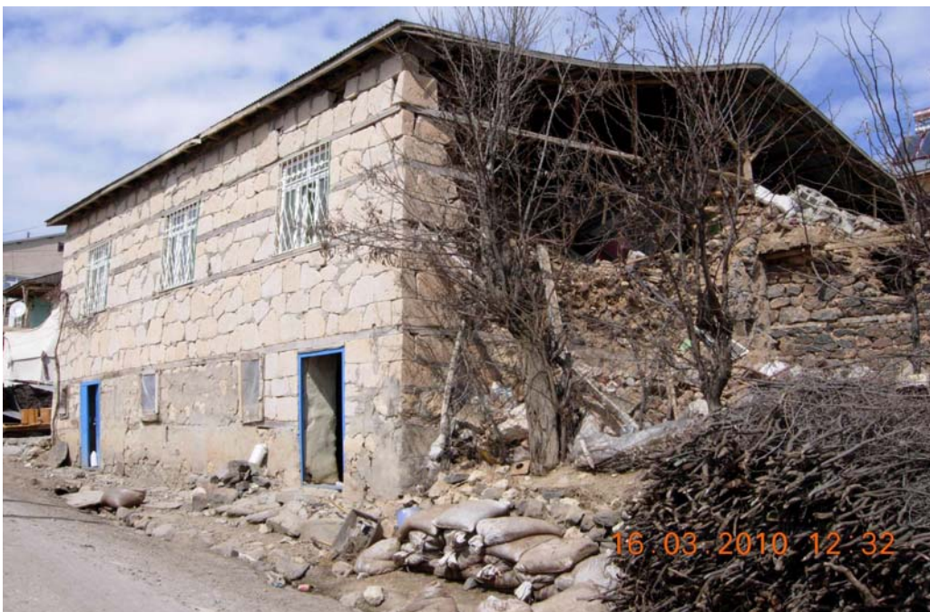
Figure 27: Two storey light stone house, with a stall as ground floor, Okcular village
