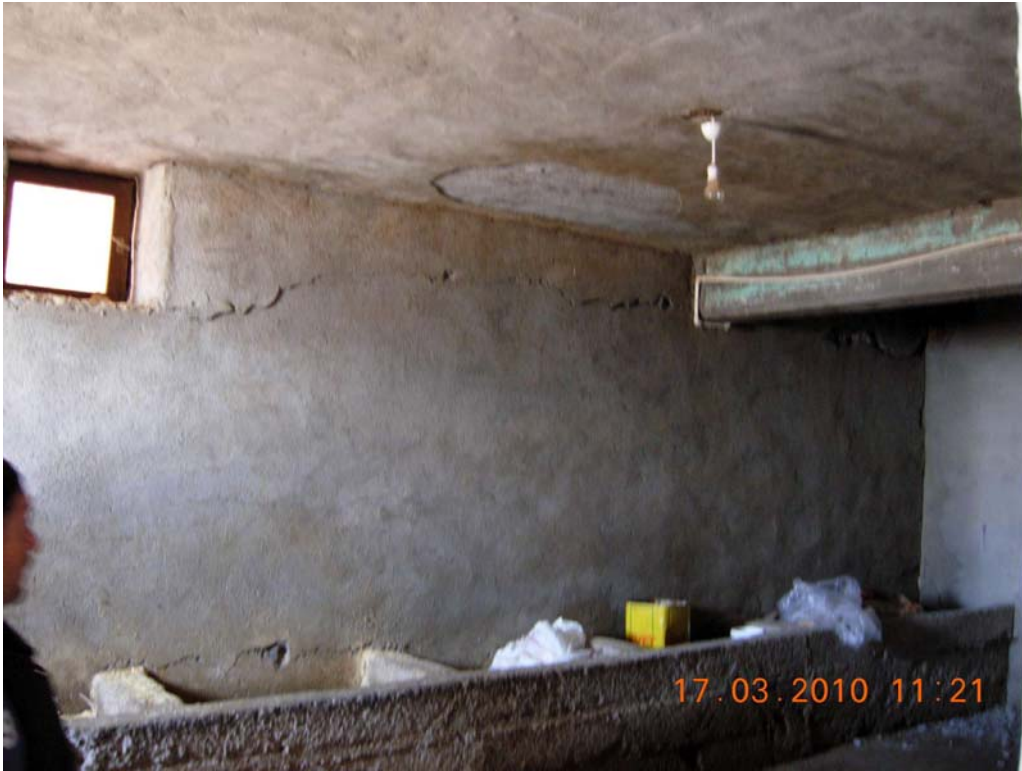
Figure 41: Inside view of two storeys mixed structural system, RC beam, RC slab, heavy stone wall, Okular village
