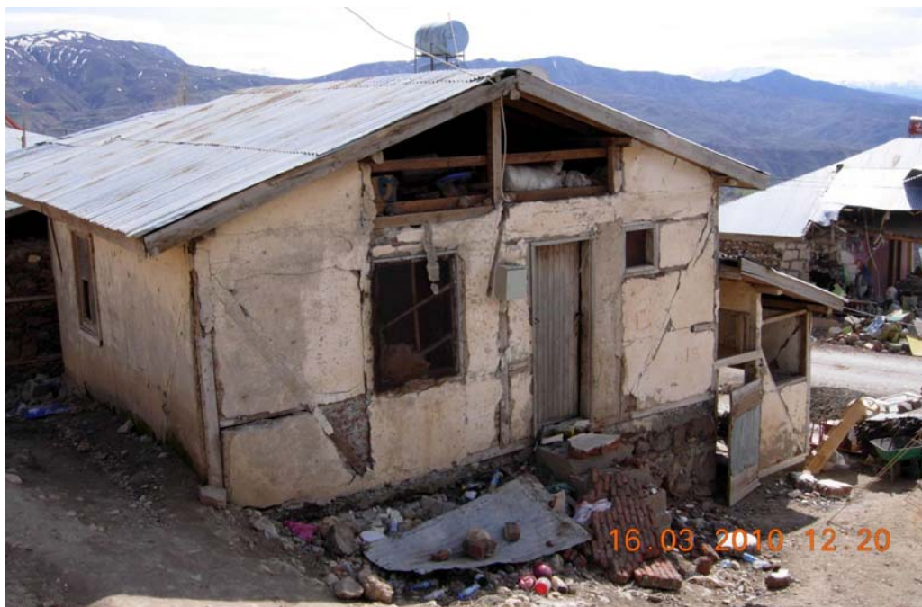
Figure 58: Refractory brick houses built after 1971 Bingol earthquake, Okcular
