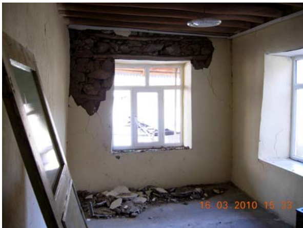
Figure 83: Wide cracks around openings, Beyhan-Palu
