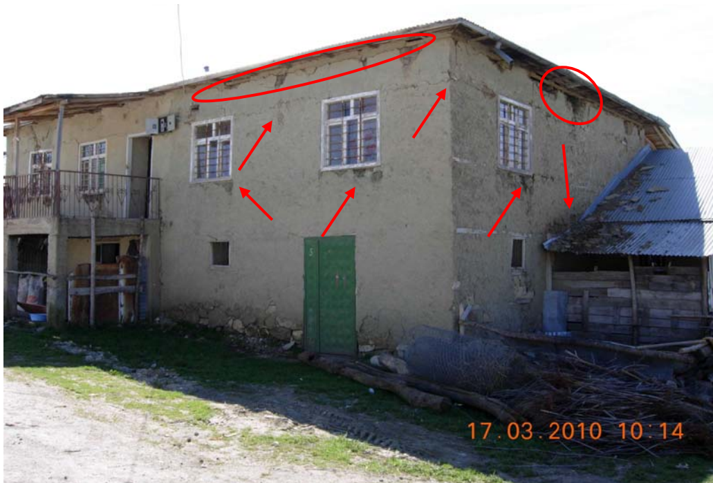
Figure 22: Two storey soil brick house in Incedal village-front view
