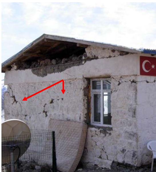
Figure 81: Wide cracks following the mortar, school building side view, Kayalık village
