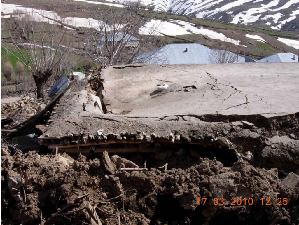
Figure 78: Thick soil layer on the roof, Kayalık village
