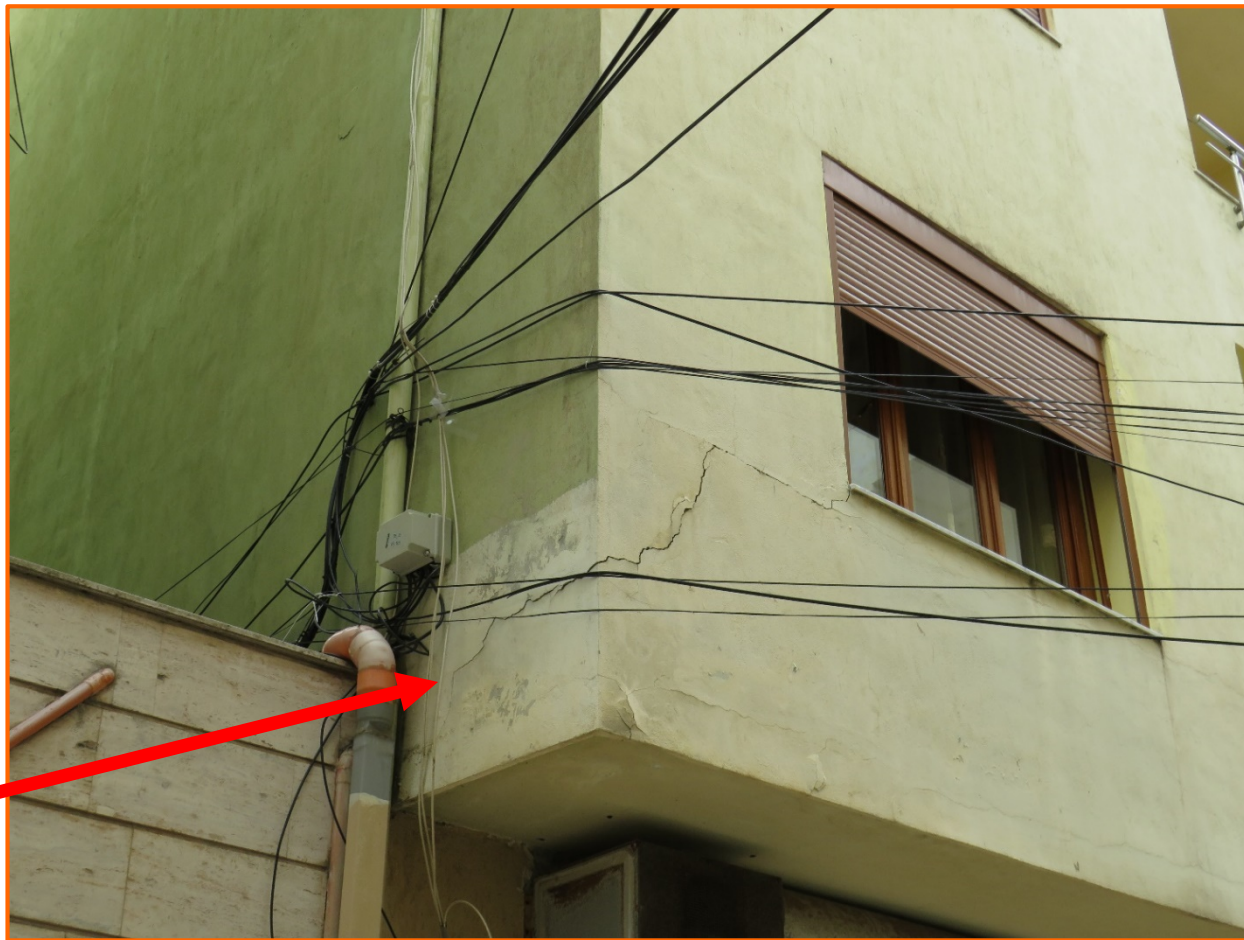
Effect of the vertical shaking component on the brick wall standing on the RC cantilever (that is excited vertically)
