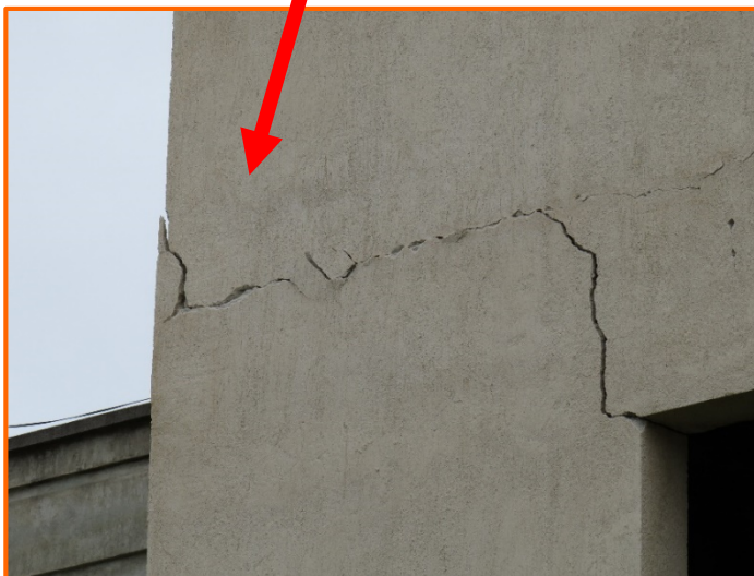
Effect of the vertical component of the earthquake ground motion in combination with the horizontal one on brick walls on an RC cantilever.
