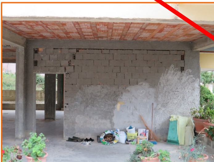
Separation of the infill brick walls from the R/C framing system
