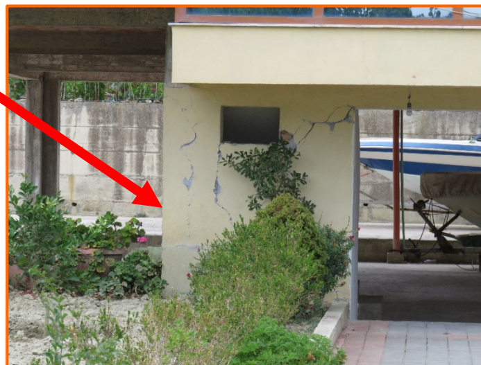
Separation of the infill brick walls from the R/C framing system
