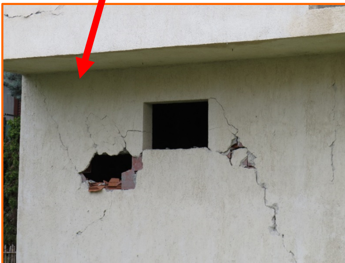
Effect of the vertical component of the earthquake ground motion in combination with the horizontal one on brick walls on an RC cantilever.
